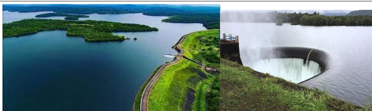
Figure 1: Salaulim Dam Reservoirs
